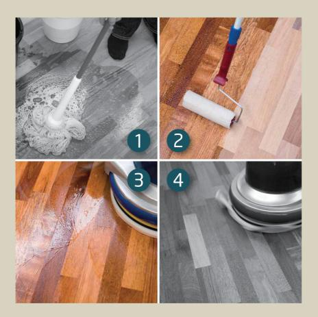
A polishing machine with beige polishing pad. Paintroller and cotton cloths. Clean tools with Solvent.
