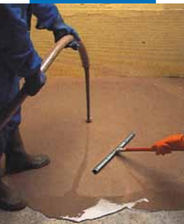
Application of Ultraplan with pump and squeegee
