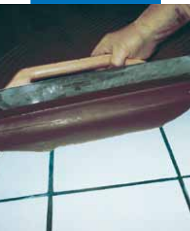
Application of Ultraplan with a metal trowel on an existing ceramic tile floor after the application of Mapeprim SP
