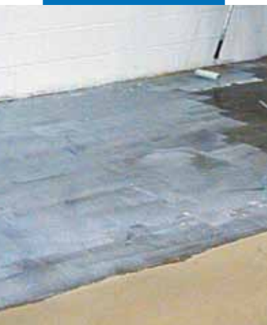
Application of Mapeprim SP
